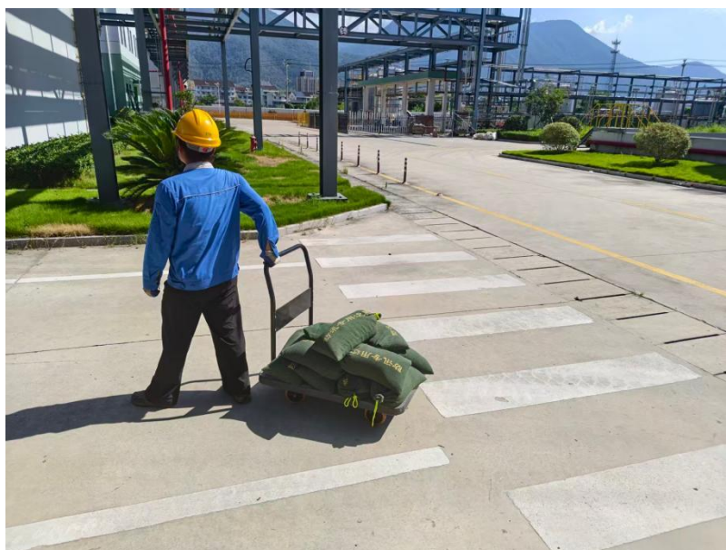
泄漏点沙袋封堵
